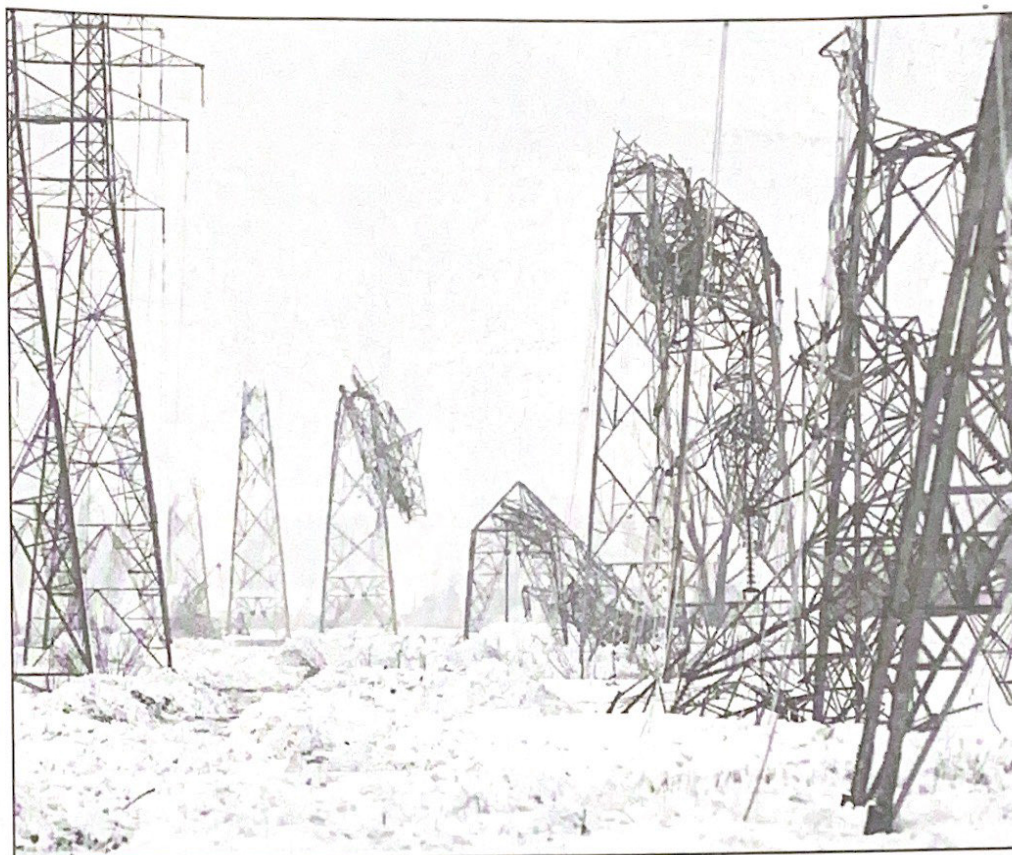
Crumpled transmission line towers sit between St. Jean-Baptiste and Marieville, Quebec, waiting for repair or replacement. The ice storm brought up to 6 inches of ice, exposing weaknesses in Hydro Quebec's power system.
