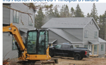
Photos: Construction continues in Stonington
