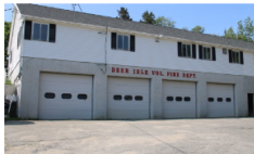
Deer Isle fire station project at a standstill until funding is found
